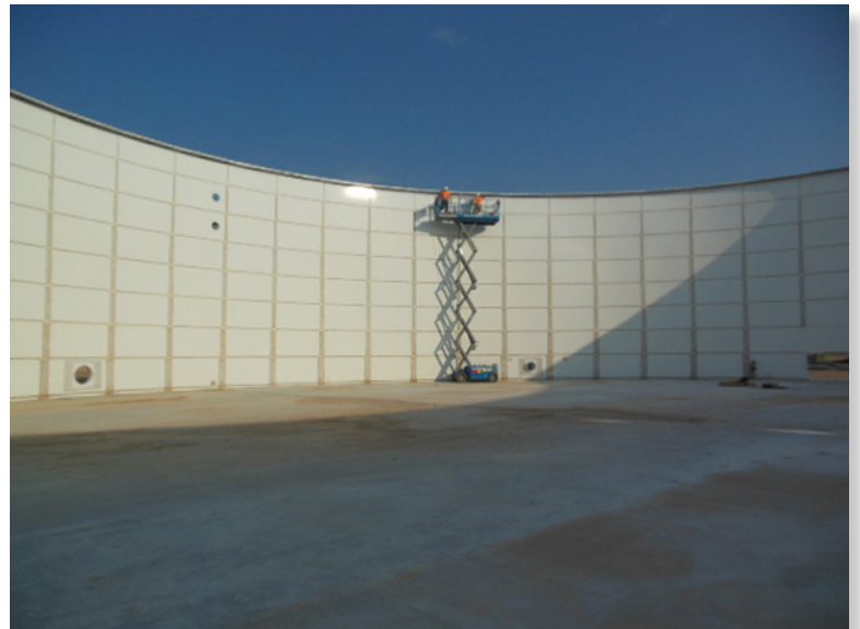
Bolted RTP Tank/Lake @ 6 Million Gallons
