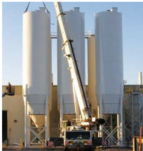
Shop-weld – ship as one piece units
