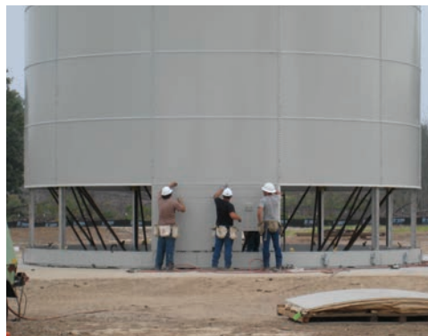
Bolted RTP Silos install from grade level
