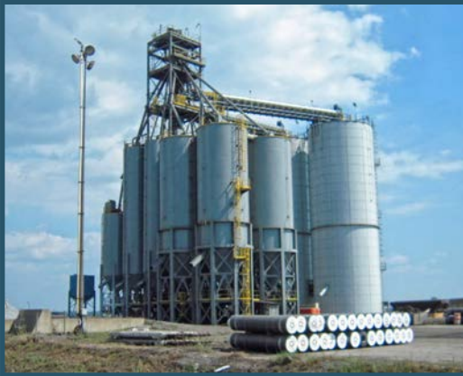
Our friends at NuCor. Picture depicts XL bolted RTP tanks by TC and field-welded tanks.
