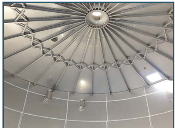
Bolted stainless steel construction available in 304L, 316 and 316L construction.
