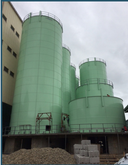
Tanks under Construction • Philippines
