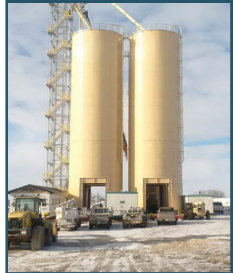
Tanks under Construction Grand Prairie, Alberta Canada
