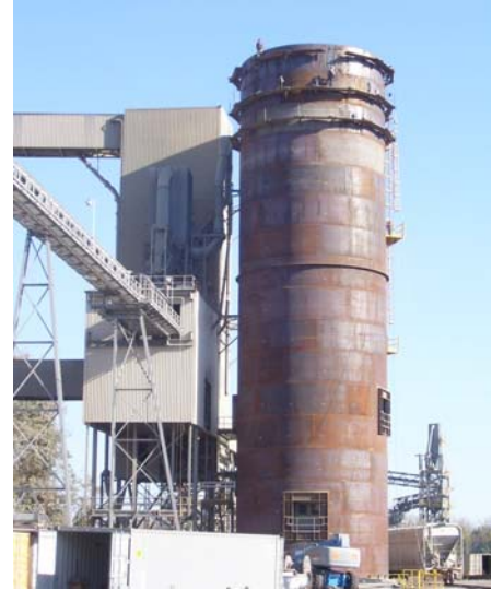
Field-weld construction
