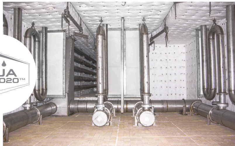
Advanced continuous furnace technology
