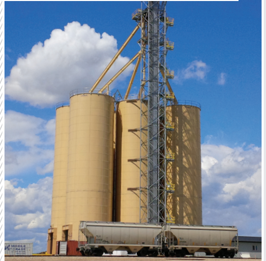
RTP (rolled, tapered panel) bolted design
