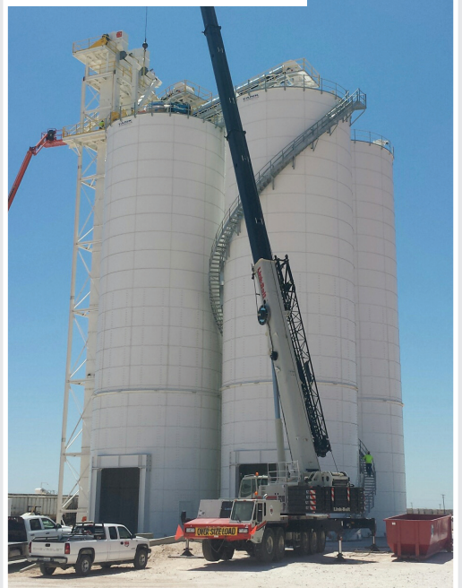
RTP tank under construction
