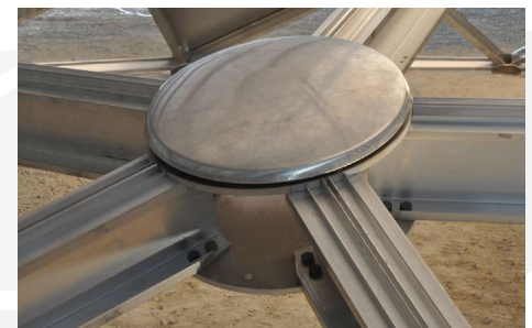
Competitor Design - Pressed cover provides inconsistent seal.
