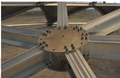
Node detail utilizes proprietary extrusion design.
