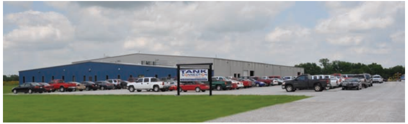
Another Tank Connection manufacturing facility was unveiled in December 2008. Facility manufactures the top rated "RTP" bolted tank design selected worldwide.
