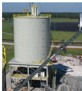
Bolted RTP - Process Storage
