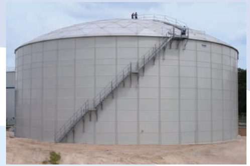
RTP Construction - Pure Water Storage 4.5 million gallons/ 17,000 m 3
