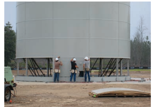
Standpipe - jacked from grade level
