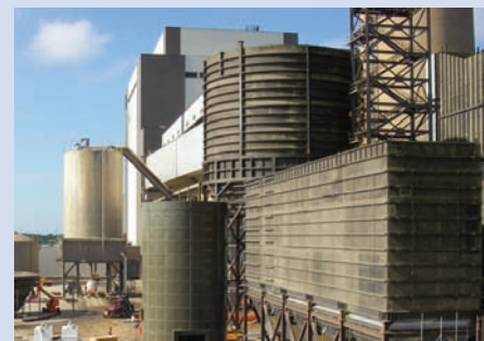
Bolted RTP, Field-weld & Hybrid Tank Construction
