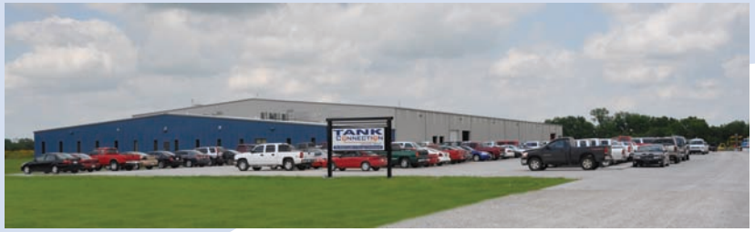
Another Tank Connection manufacturing facility was unveiled in December 2008. Facility manufactures the top rated "RTP" bolted tank design selected worldwide.
