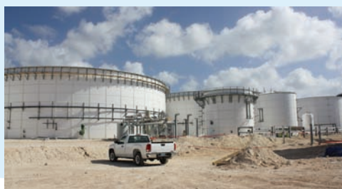
Water & Wastewater Facility
