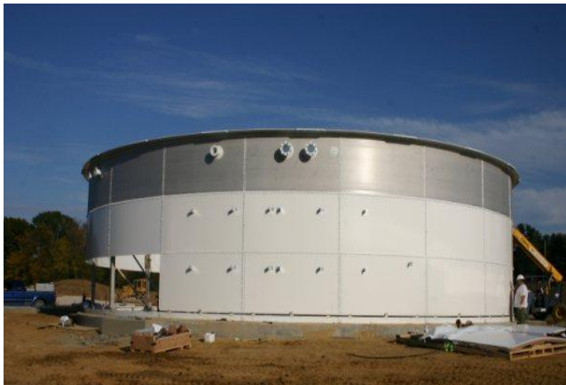
Hybrid digester tank under construction
