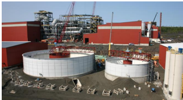
Clarifiers Bolted RTP Hybrid Construction
