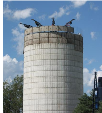
Jump-Form Pedestal For Elevated Water Tank
