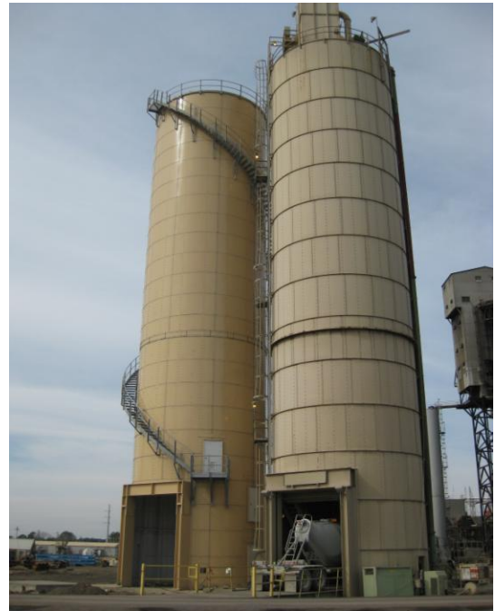
RTP (rolled, tapered panel) Construction (left) API 12B Flanged Panel Construction (right)
