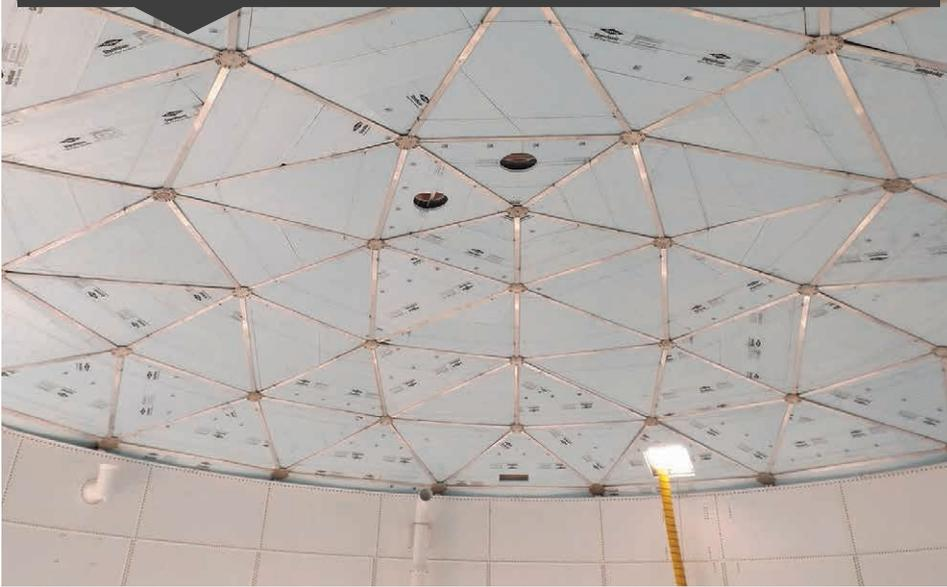
Apex Domes provides interior insulation at up to three inches in thickness. The insulation panels can be applied either on the ground during assembly or after the dome is completed.
