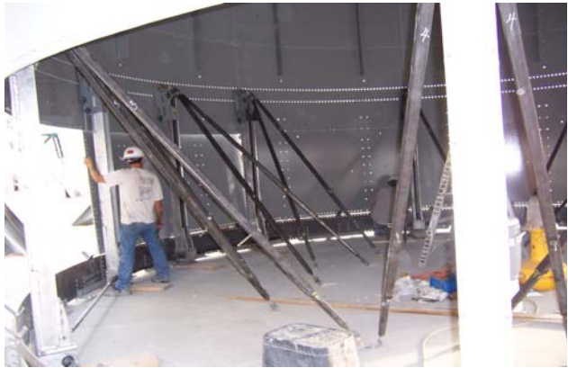
Dry Bulk Hopper Storage
