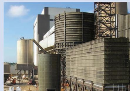
Bolted RTP, Field-weld & Hybrid Tank Construction
