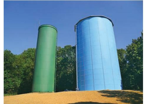
Field-Weld Standpipe      Bolted RTP Standpipe
