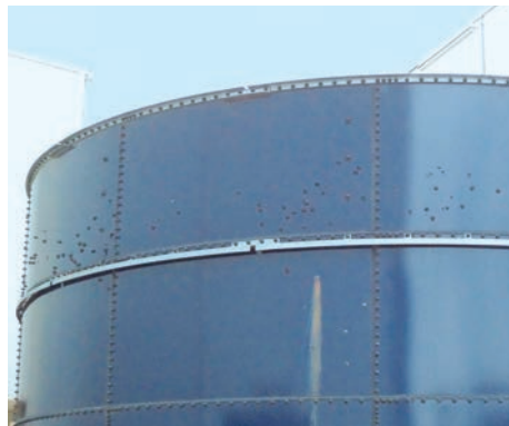
Glass coated with surface defects 10 years old
